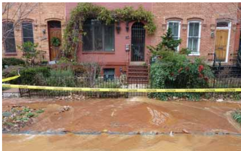
The unexpected water feature that appeared in our front yard as we were trying to get out of town. WASA came. And installed hazard tape.
