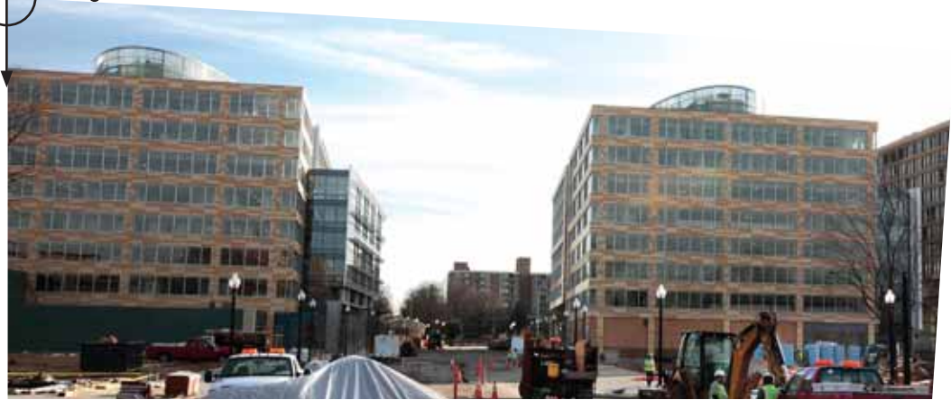
A new streetscape is taking shape along Fourth Street SW, which is a big change from a few years ago when the only direct pedestrian access from the north to the Waterfront Metro station was to walk through the old Waterside Mall. Photo: Andrew Lightman
