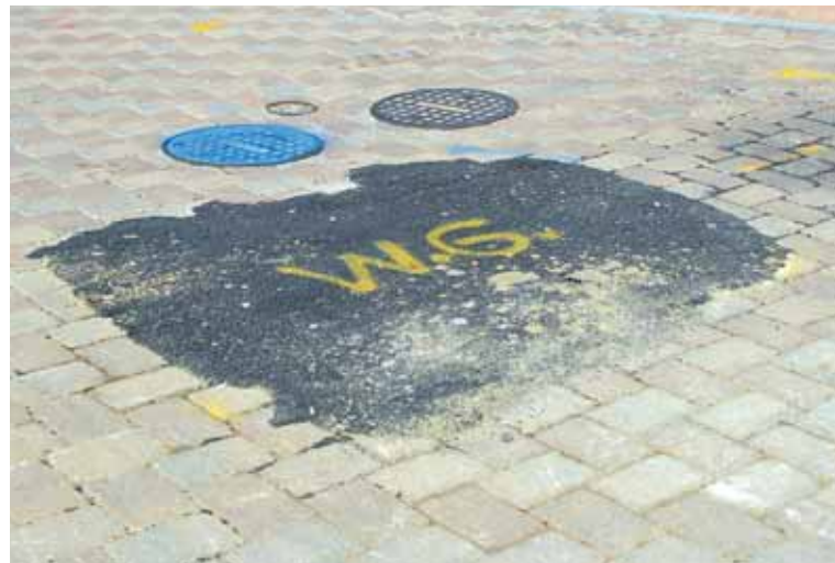
ABOVE: Rather than replacing the pavers, Washington Gas patched the street with ugly cold pack. Photo: Andrew Lightman
