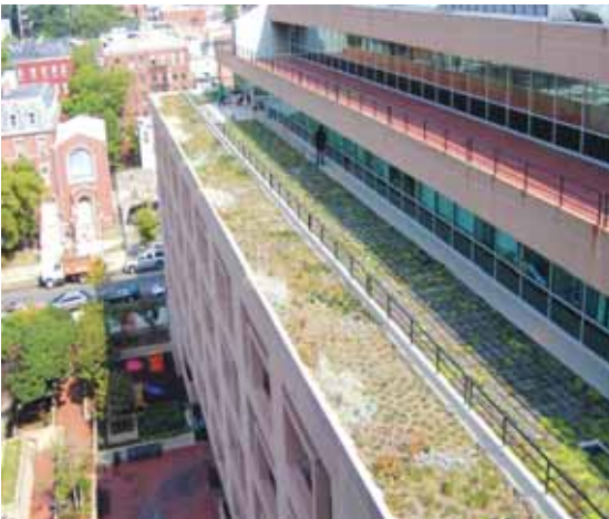
Before and after pictures of the extensive modular green roof we did at the Reeves building.
