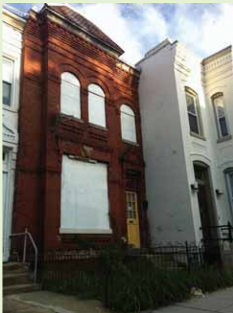
1539 9th St. is set for a major restoration and renovation and will become two condominiums. Photo: Ralph Brabham
