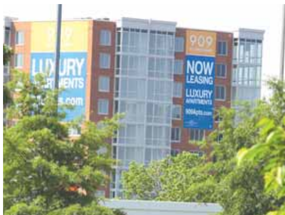
TOP: The Yards, a development of Forest City Washington. Courtesy Capitol Riverfront BID
